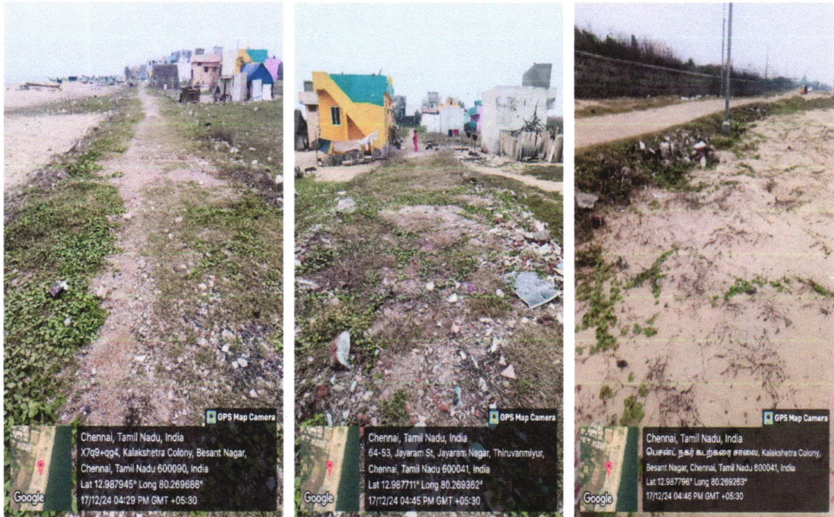
Fig 3. Three sand roads constructed near to the Arupadai Veedu Murugan Temple in Besant Nagar's Kalakshetra Colony in Chennai (Tamil Nadu)
